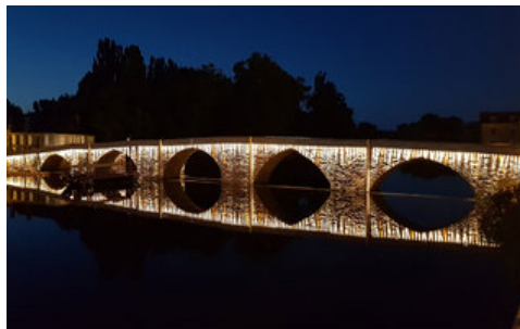
Old Bridge in Terrasson-Lavilledieu
