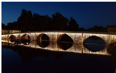
Old Bridge in Terrasson-Lavilledieu
